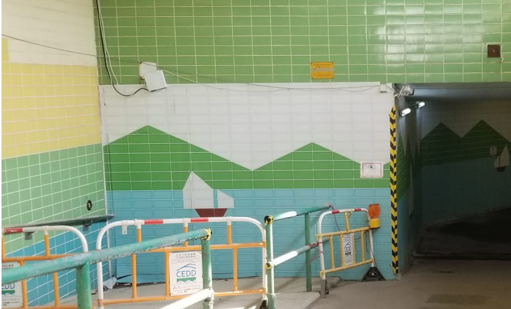
Photo 3 – Erection of site hoardings in unobtrusive colours
