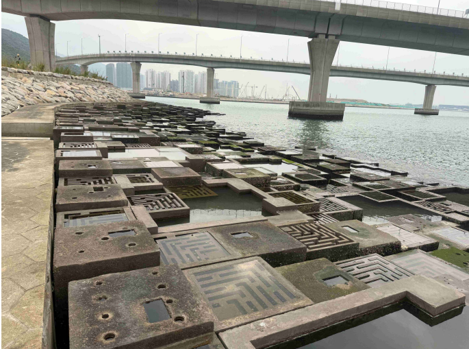
General View of Rocky Eco-shoreline
